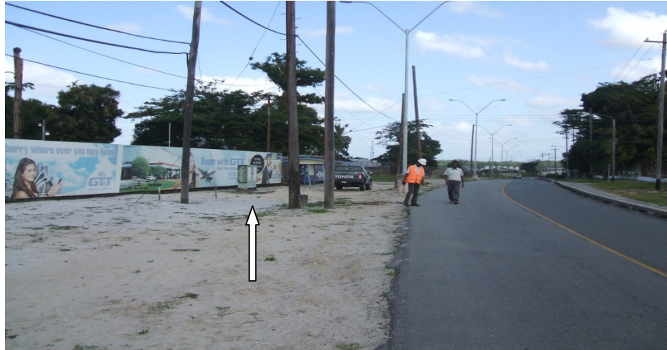
Fig. 4 - Poles and junction box in path of roadway (February 2014)
