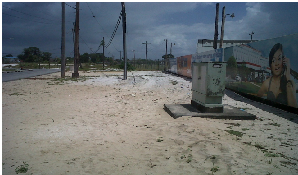
Fig. 3 - Poles & junction box in path of the road construction (March 2013)
