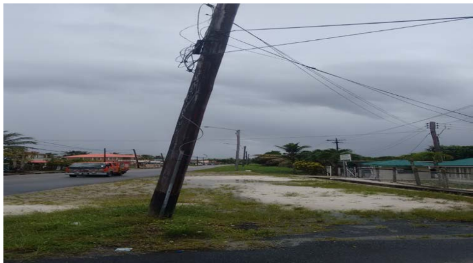
Fig. 6 - Utility pole in path of incomplete roadway (15 September 2016)
