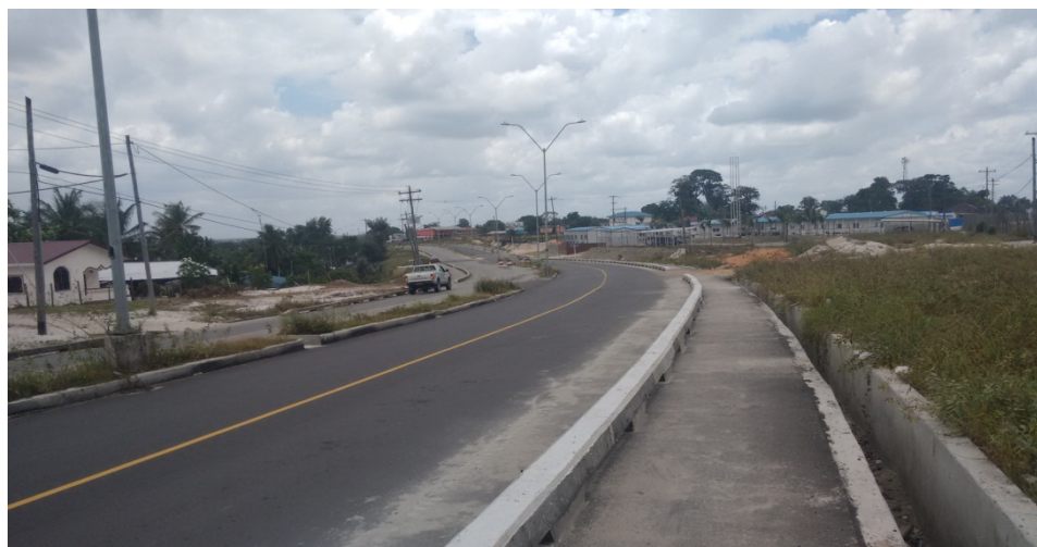
Fig. 5 - New Access Road substantially completed (March 2016)
